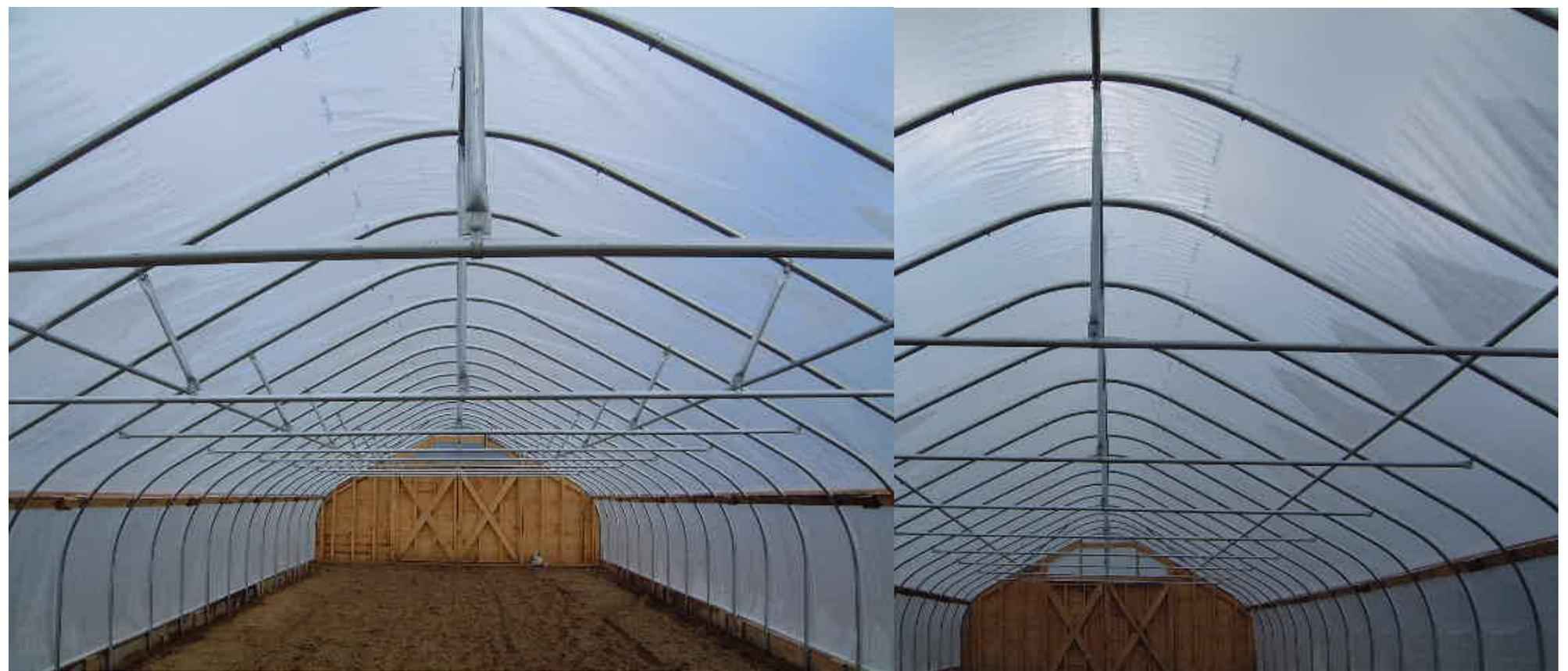
Connect the drop to the crosstie using two small clamps. One attached to the ridge purlin and the other around the crosstie.
