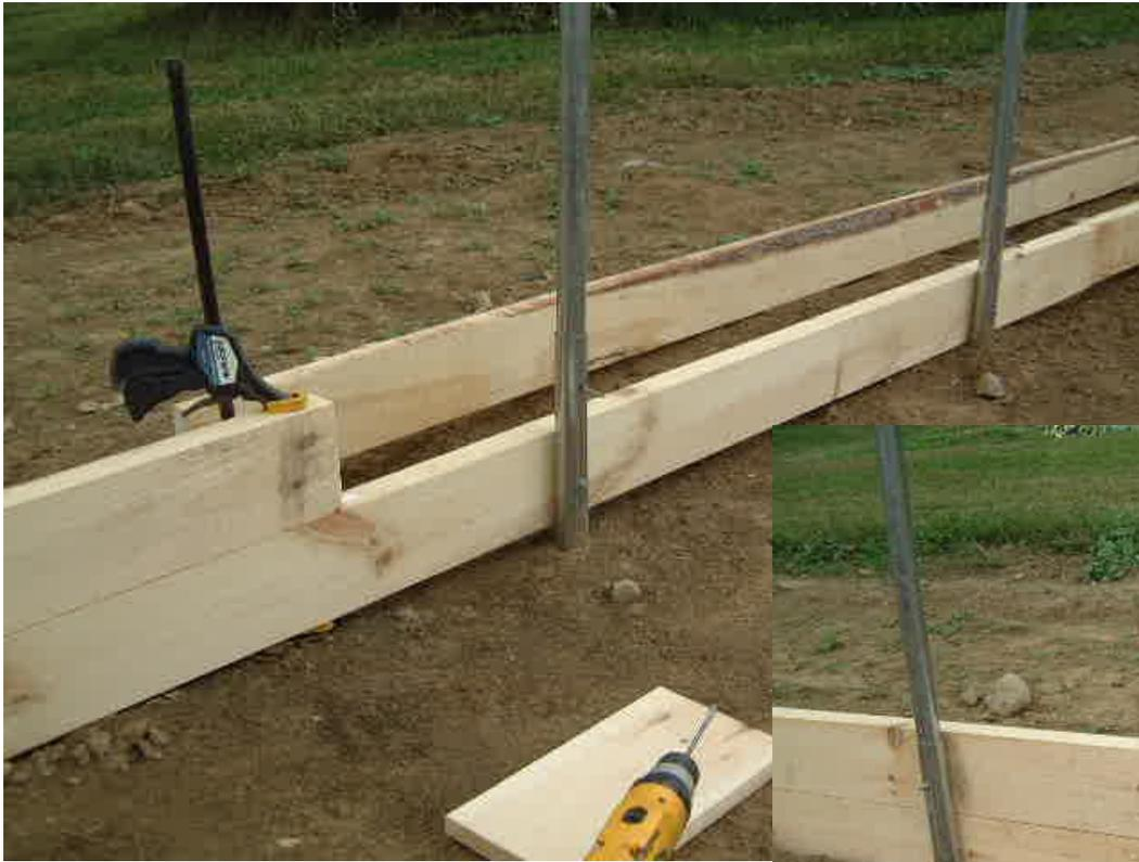
Use a second layer or one wide plank. Connect the joints with pieces of board.
