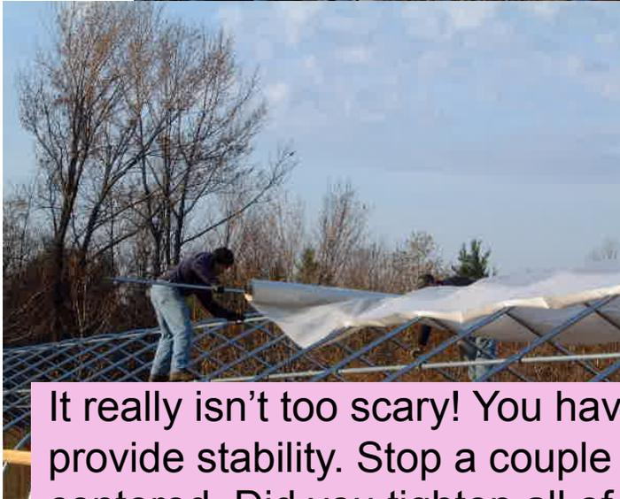
It really isn't too scary! You have the roll, the long pipe and your most trusted to provide stability. Stop a couple of times to pull the roll tight and make sure it is centered. Did you tighten all of the bolts?
