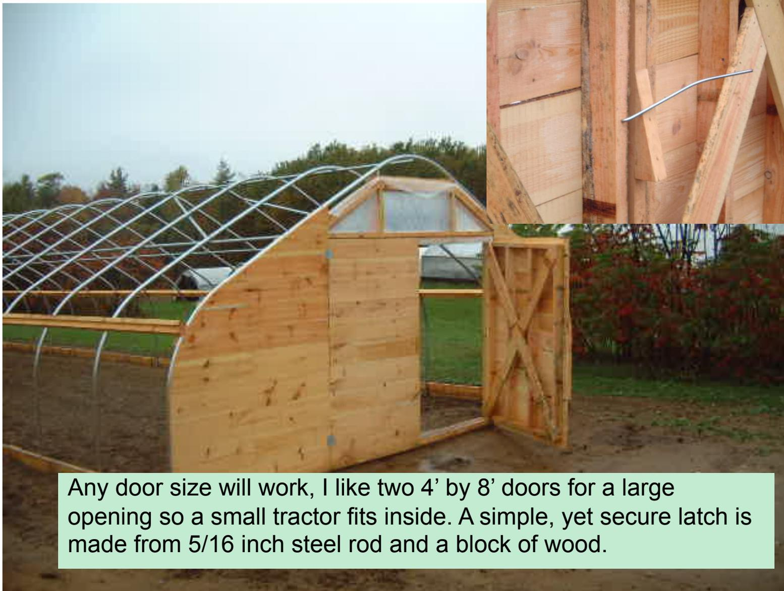
Any door size will work, I like two 4' by 8' doors for a large opening so a small tractor fits inside. A simple, yet secure latch is made from 5/16 inch steel rod and a block of wood.
