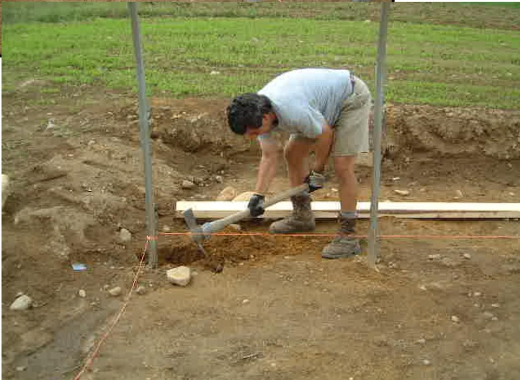
Dig the soil out of the way so the top of the board will line up with the marks on the posts.
