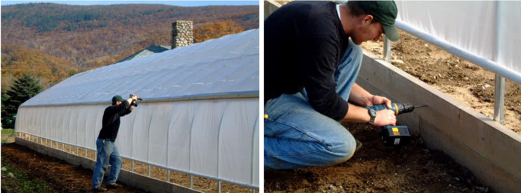
Attach the bolts or eyes about midway between two bows. The bottom bolt will be about 3" below the top of the baseboard and the top bolt through the poly cleat. The ropes will be located every other bow, starting at the end bow.
