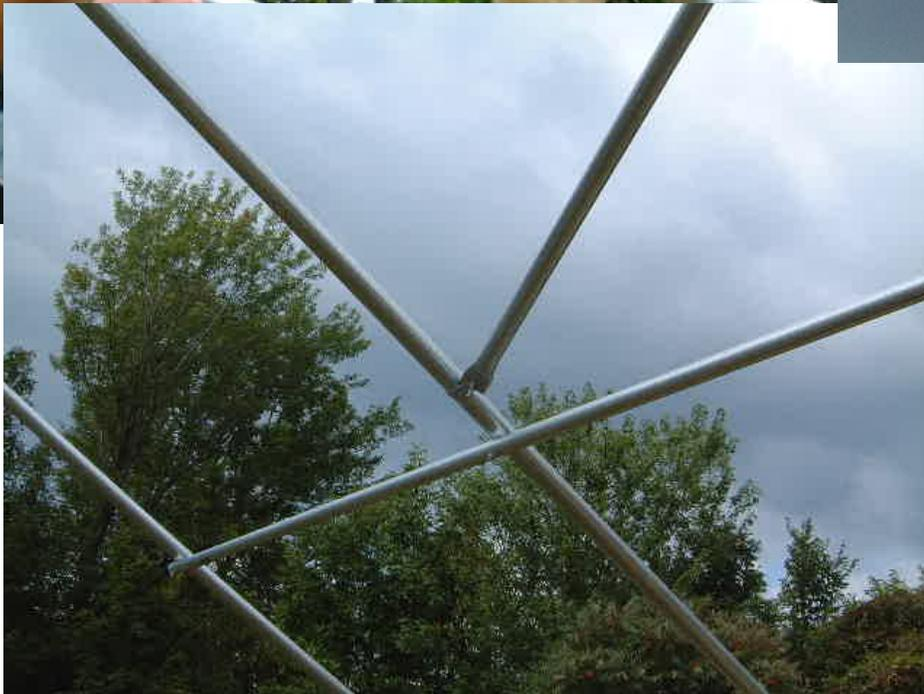
Clamp the lower end of a corner brace to the second bow using a long clamp, then pivot the corner brace so the other end can be clamped to the fourth bow with another long clamp.
