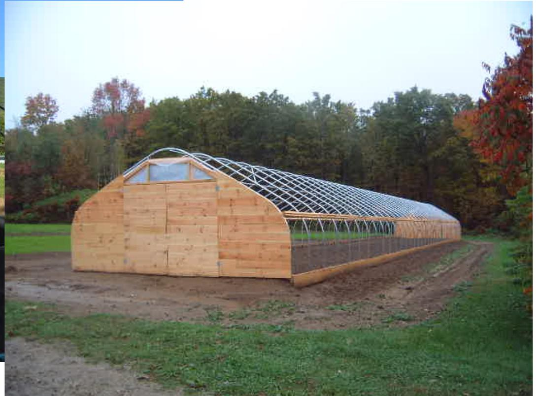
You may use any material to finish the ends. Poly, clear structured sheets, boards, or plywood. I often use plywood as it is fast and durable.
